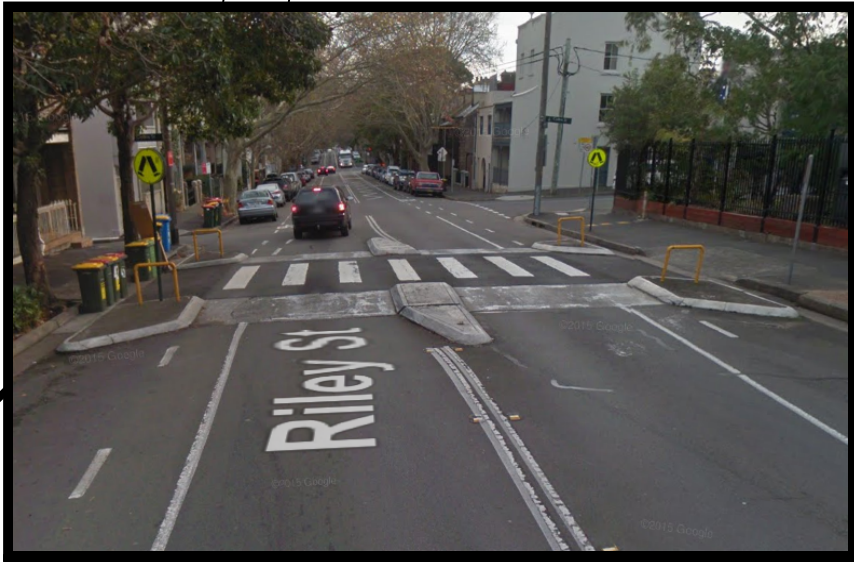
EXISTING CROSSING REQUIRES ADJUSTMENT TO SUIT NEW PARKING LAYOUT . IMAGE SOURCE: GOOGLE MAPS STREET VIEW
